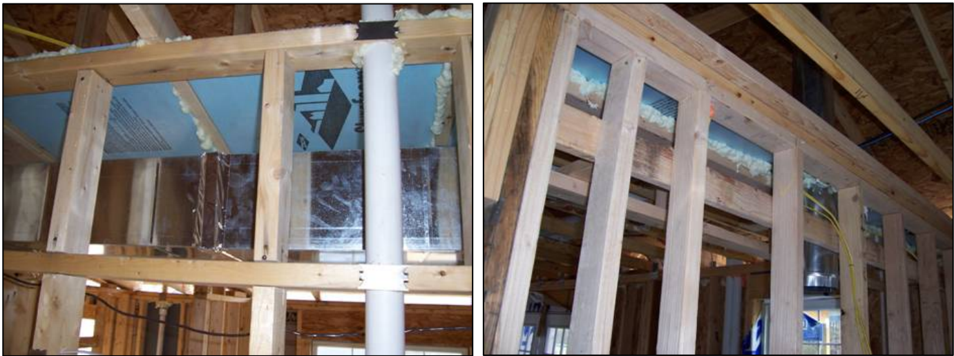
Figure 5.3.4 - Air sealed soffits
