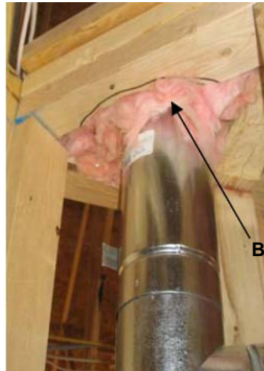
Figure 4.3.1 - Insulation improperly used as an air barrier
