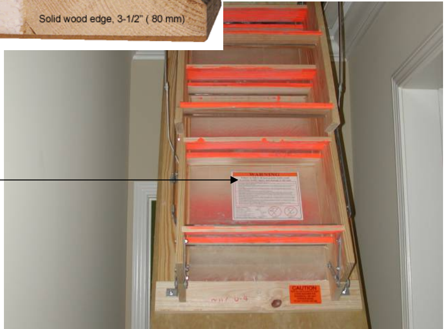
Figure 5.2.3 – Pre-insulated/sealed attic drop-down stair assembly
