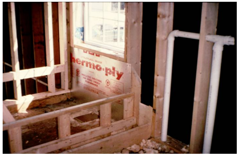
Figure 2.1.3 – Architectural detail of tub installation with complete air and thermal barriers
