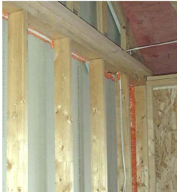
Figure 6.1.4 - Example of properly air sealed common wall with fire-rated caulking (in red)
