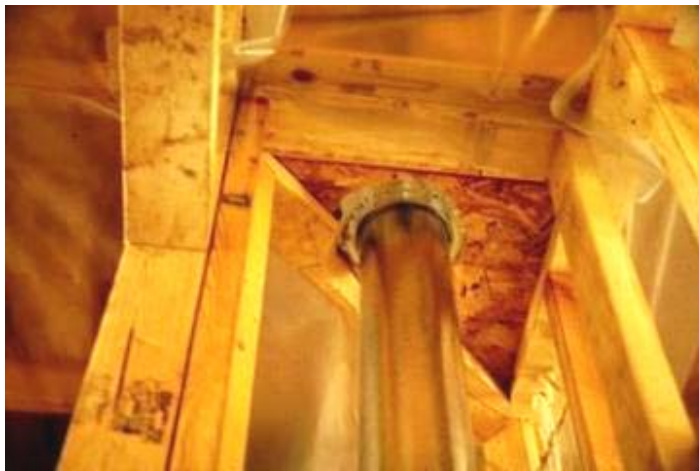
Figure 4.3.2 - UL-rated metal collar installed around a flue shaft
