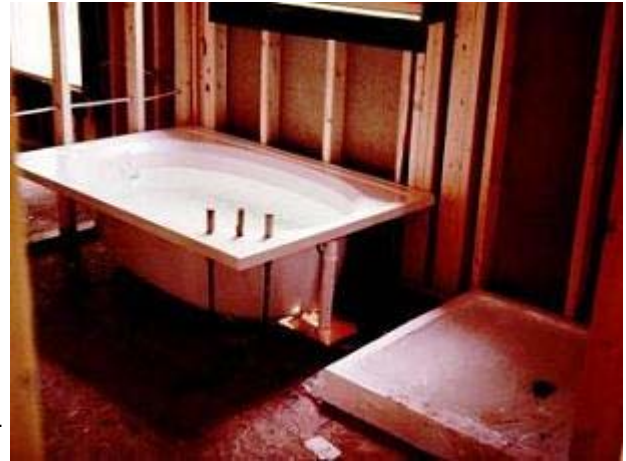
Figure 2.1.1 - Tub installed against exterior wall without air barrier or insulation
