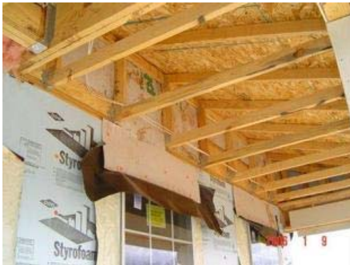
Figure 2.6.4 - Appropriate blocking between sloped porch roof and conditioned space
