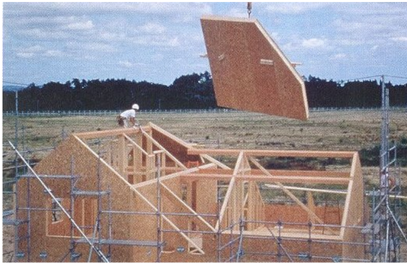
Figure 1.6.4 - Structural Insulated Panels (SIPs)
