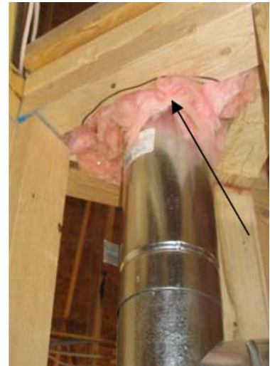
Figure 4.1.2 – Duct shaft with ineffective air barrier (insulation)
