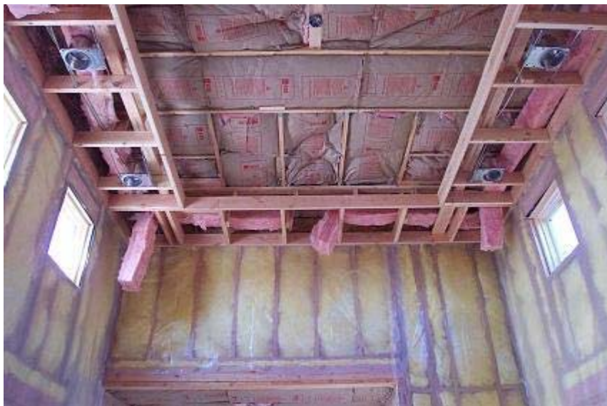
Figure 5.3.1 - Improperly installed insulation over a dropped ceiling
