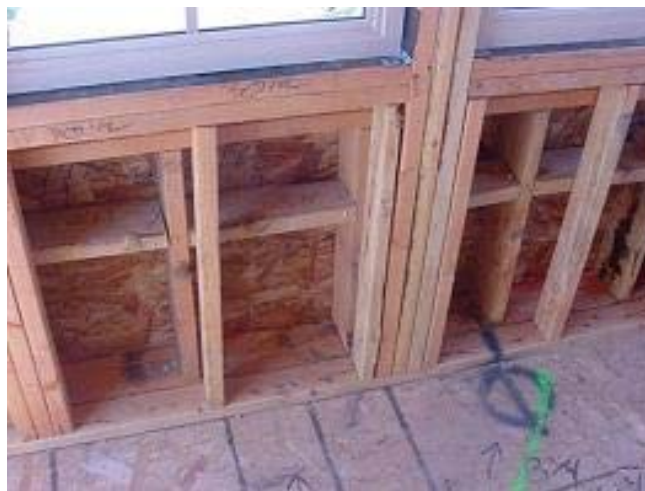
Figure 2.8.3 – Example of a double wall
