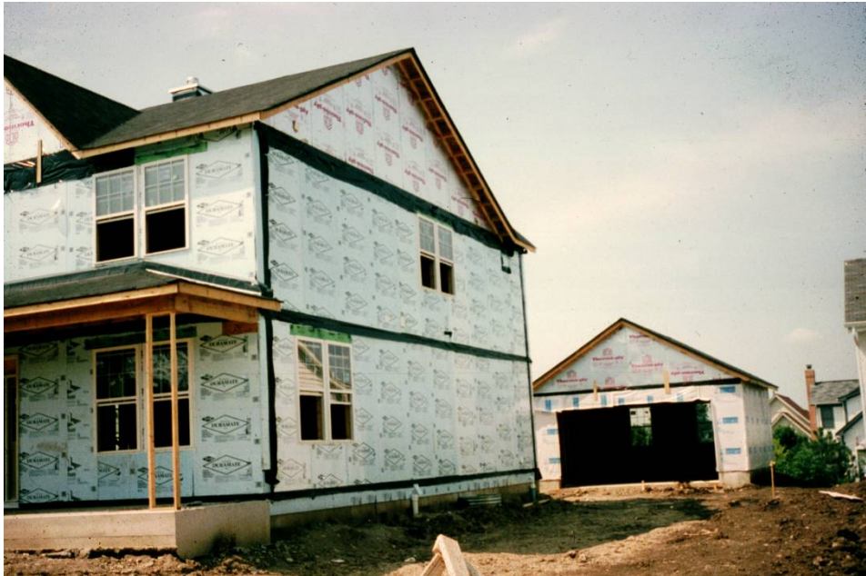
Figure 1.6.3 – Complete thermal break with rigid insulation sheathing
