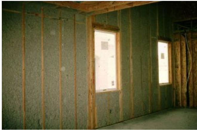
Figure 1.1.9 - Blown cellulose insulation
