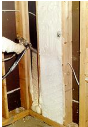
Figure 1.1.10 - Spray foam insulation
