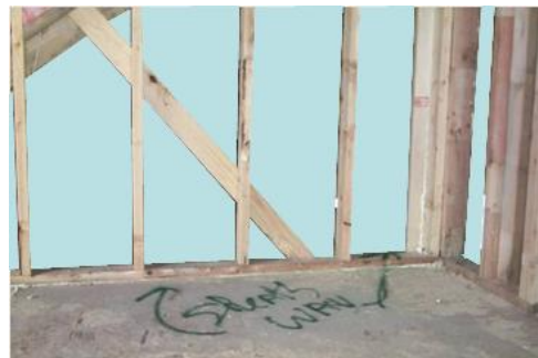
Figure 2.4.5 – Attic knee wall with exterior air barrier
