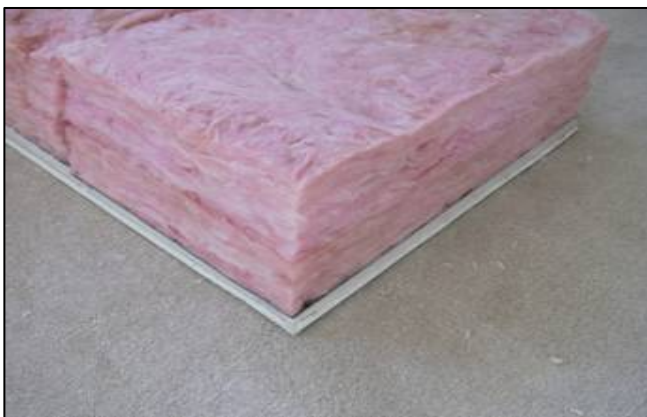
Figure 5.1.2 - Example of properly insulated and sealed attic hatch
