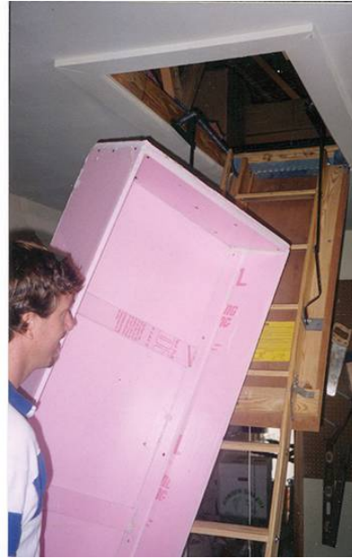
Figure 5.2.3 - Option for insulation of drop-down stair
