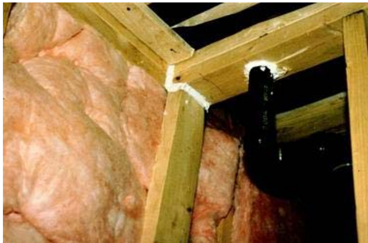
Figure 4.2.2 - Caulking around piping penetration
