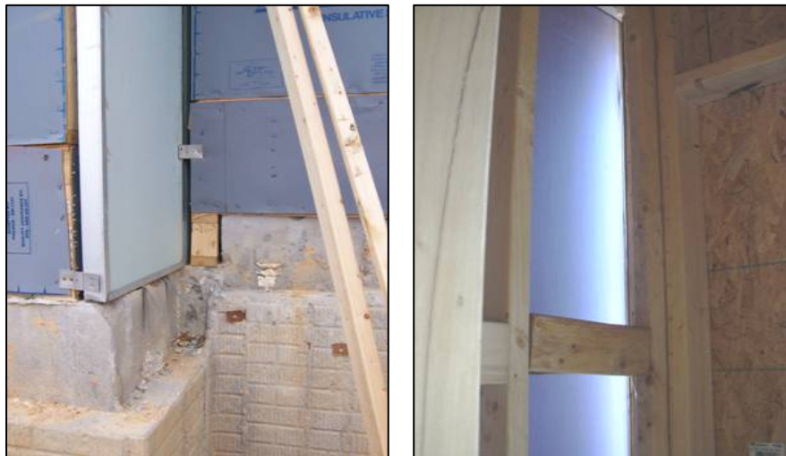
Figure 6.1.2 - Poorly sealed common wall
