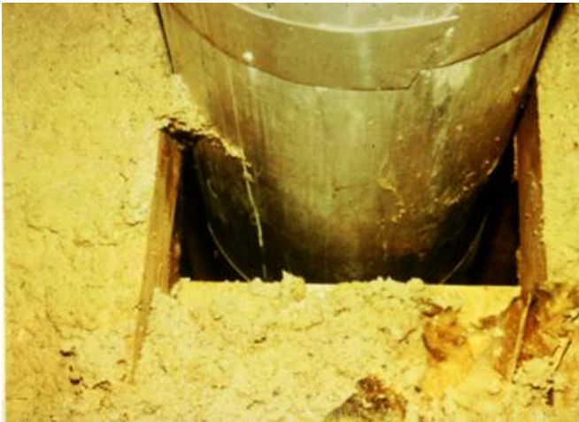
Figure 4.1.1 – Duct penetration to attic that needs blocking
