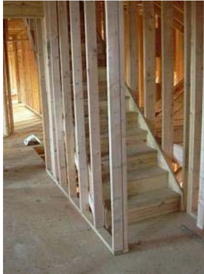
Figure 2.7.1 - Staircase adjoining unconditioned attic needs to be fully blocked and sealed
