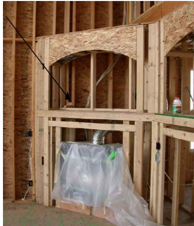
Figure 2.2.1 - Fireplace installed without air barrier
