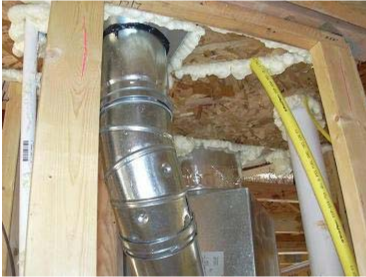
Figure 4.1.4 - Blocking and foam air sealing in chase
