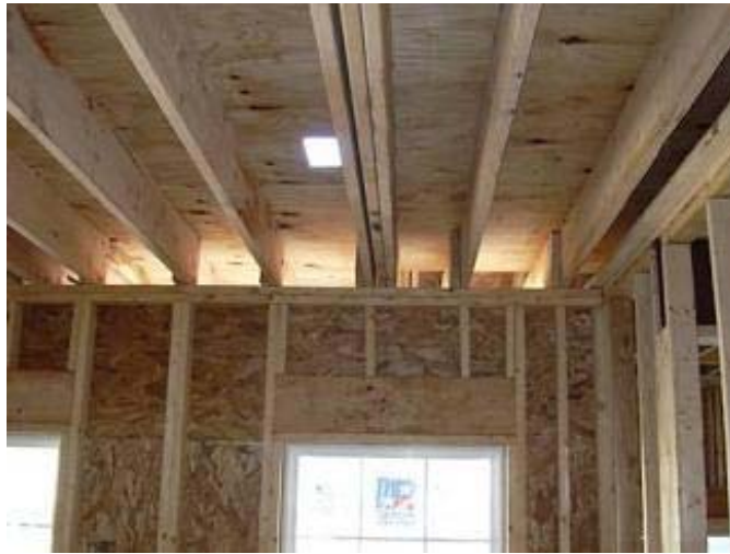
Figure 2.6.1 – Air barrier missing at porch roof
