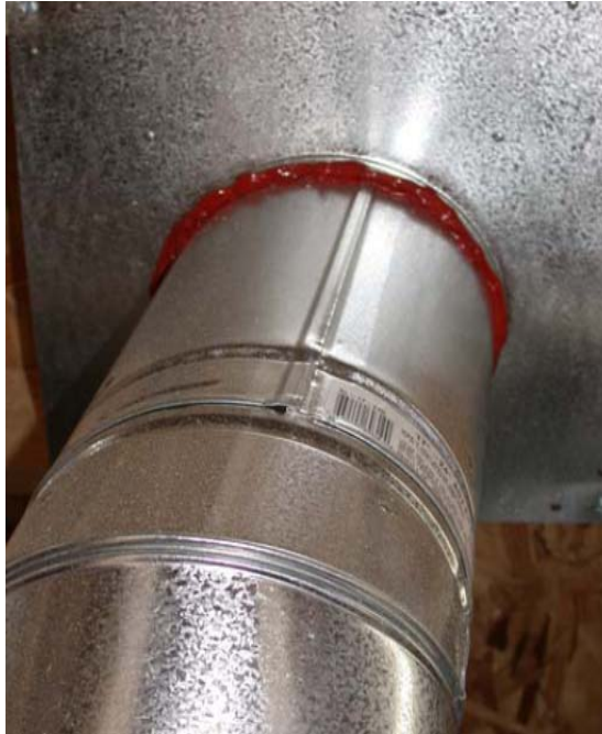
Figure 4.3.3 - Fire-rated caulk around a flue shaft
