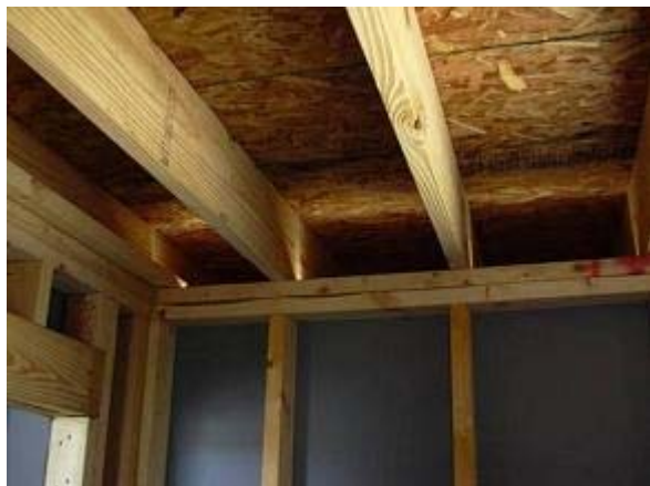
Figure 3.2.1 – Cantilevered floor with no air barrier between overhang and conditioned space
